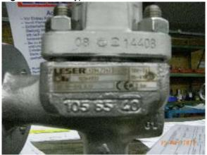
**Figure 6.2.1-6:** Standard plate on a flanged valve
