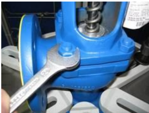
Fig. 1 Unscrewing a screw connection
