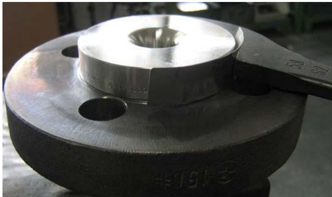
Fig. 3 Installing the nozzle
