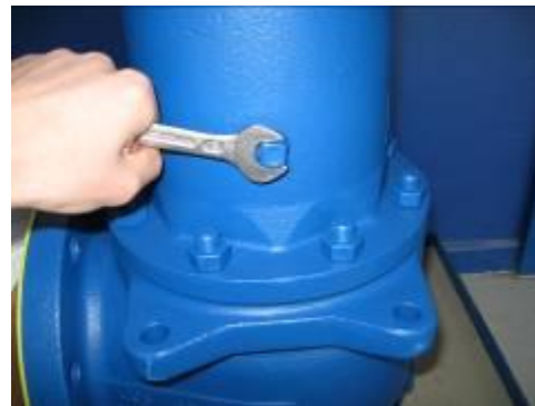
Fig. 2 Sealing the drain hole
